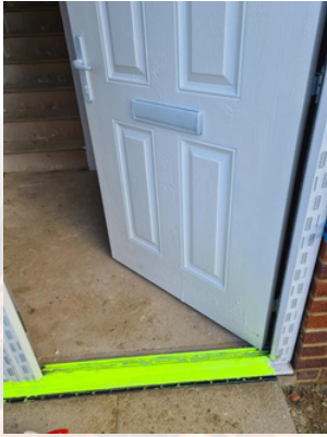
Front entrance threshold step
